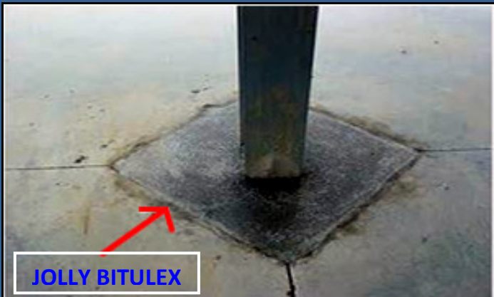
JOLLY EXPANSION JOINT FILLER IN COLUMN JOINTS
