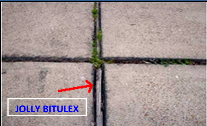
JOLLY EXPANSION JOINT FILLER IN SIDE WALK
