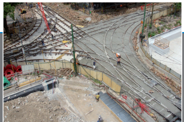
Example of foundations reinforced with concrete fibre-reinforced with iBETON 39
