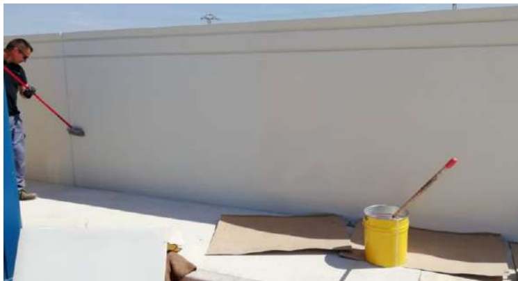
SIKA AT WORK FACTORY PERIMETER WALL – VALENCIA, SPAIN.
